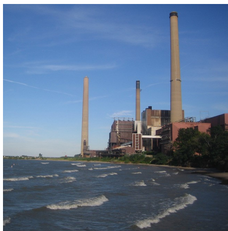
Avon Lake power plant
