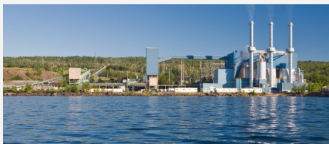
Taconite Harbor power plant
